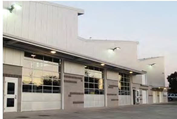
MTA Maintenance Facility. Source: LSC Transportation Consultants, Inc.
